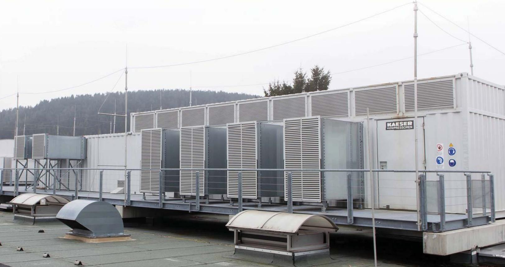
Our modified ISO shipping containers are built for easy transport and ruggedness. They can be permanent installations, but are ideal for rental installations, construction sites, or other situations where a temporary source of compressed air might be needed.
